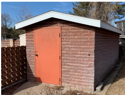
Brick Storage Shed
